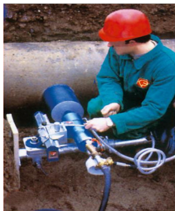
Figure 08: carottage horizontal [11]
