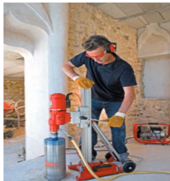
Figure 07 : carottage vertical [11]
