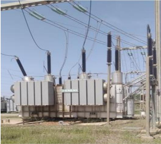
Figure II-19 : TR 220/60KV 120MVA
