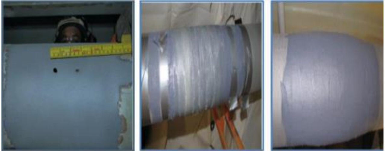
Figure 53: Composite repair of a steel pipe
