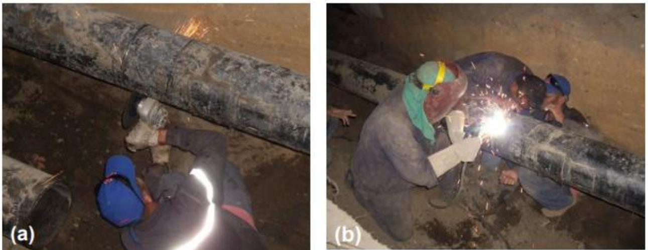
Figure 50 :Pipeline repair method
