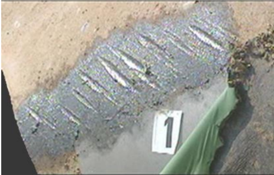
Figure 45: Example of a pipeline containing a notch [16].
