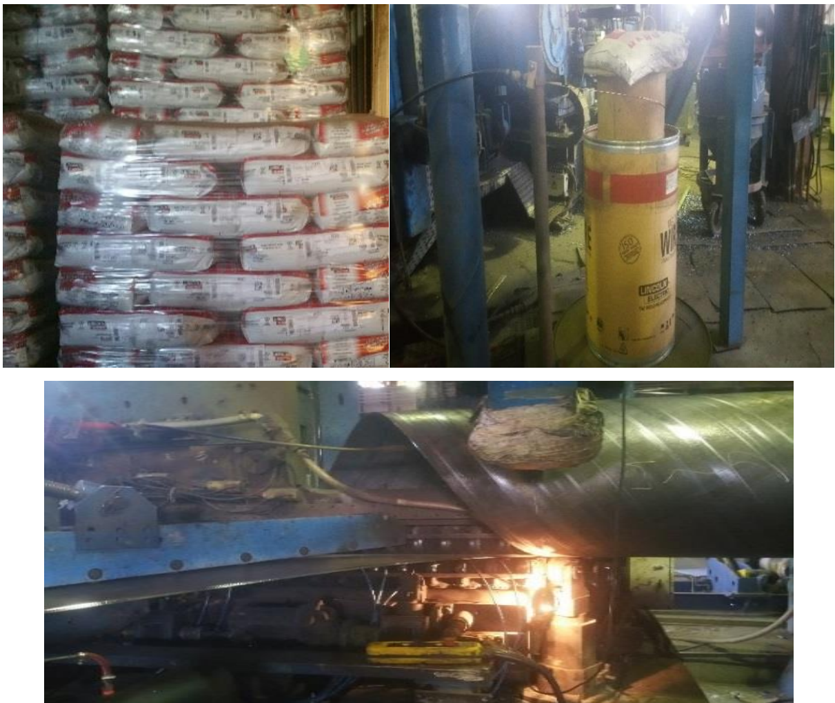
Figure 21 : interior welding of the pipe
