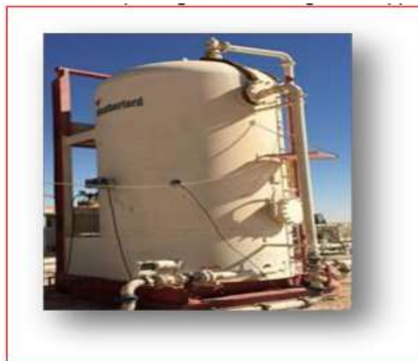
Fig 5: Mud Gas Separator
