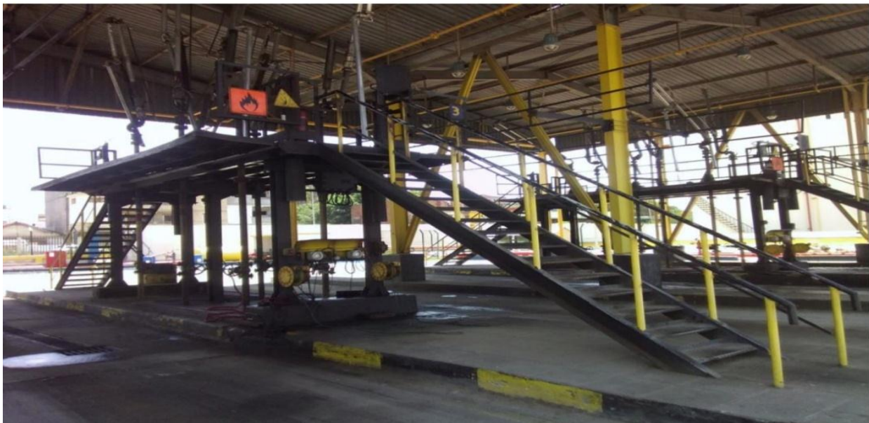
Figure IV.3: Passerelles de chargement
