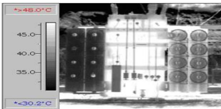
Figure 3. 15: IR for Radiators and Cooling Systems
