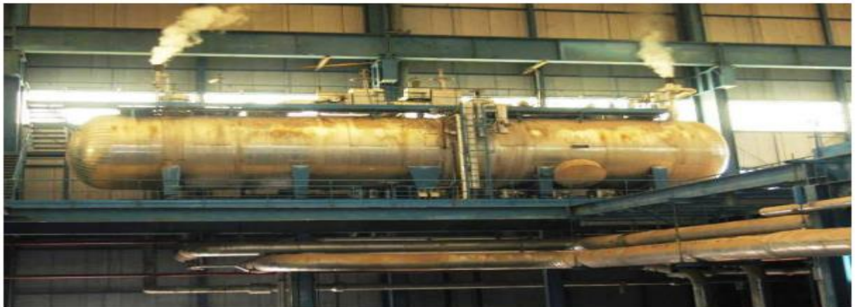
Figure 1.2-9 Feed water tank
