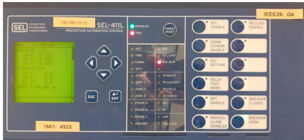
Figure 1.11: SEL-411L relay's front panel.
