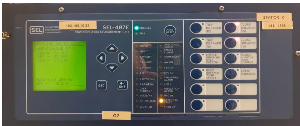
Figure 1.10: SEL-487E relay's front panel.
