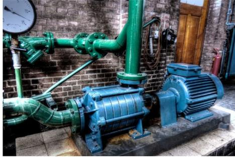
Figure I 24 pompe centrifuge
