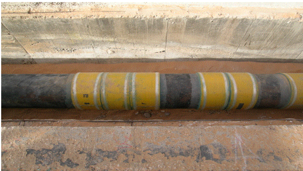
Figure III. 11: Bandes de Clock spring installées sur pipe
