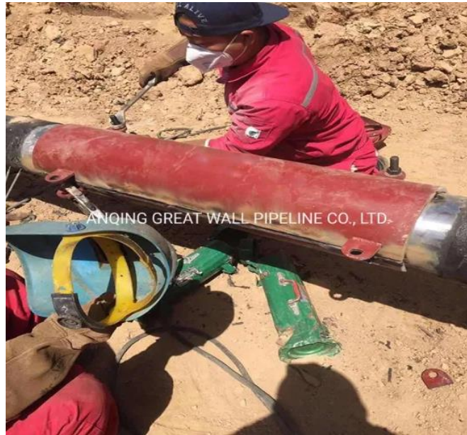
Figure III. 6 :Manchon type B
