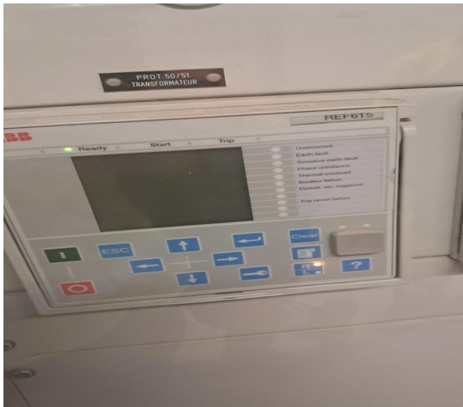
Figure 1-REF615 protective relay from ABB
