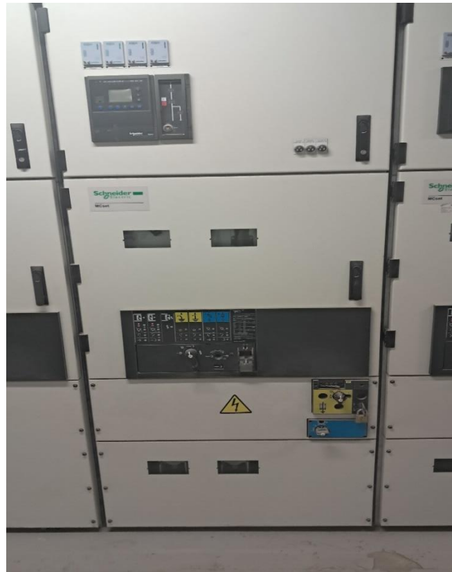
Figure 24 -medium voltage switchgear
