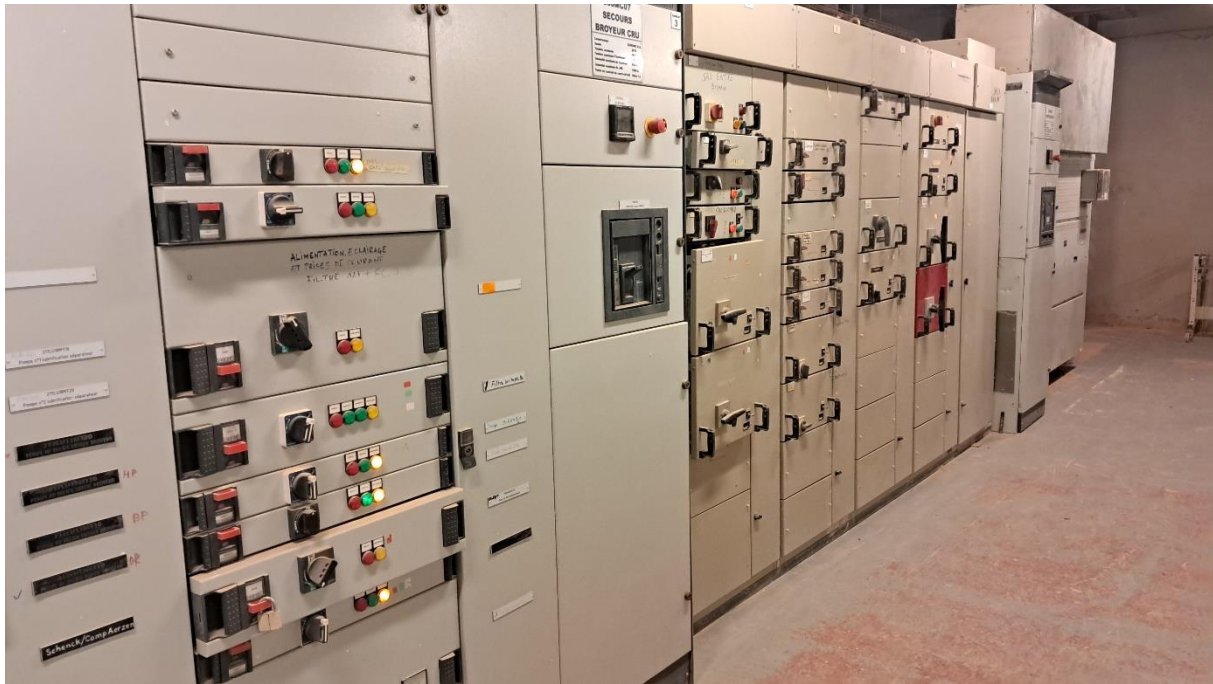
Figure 25- low voltage switchgear
