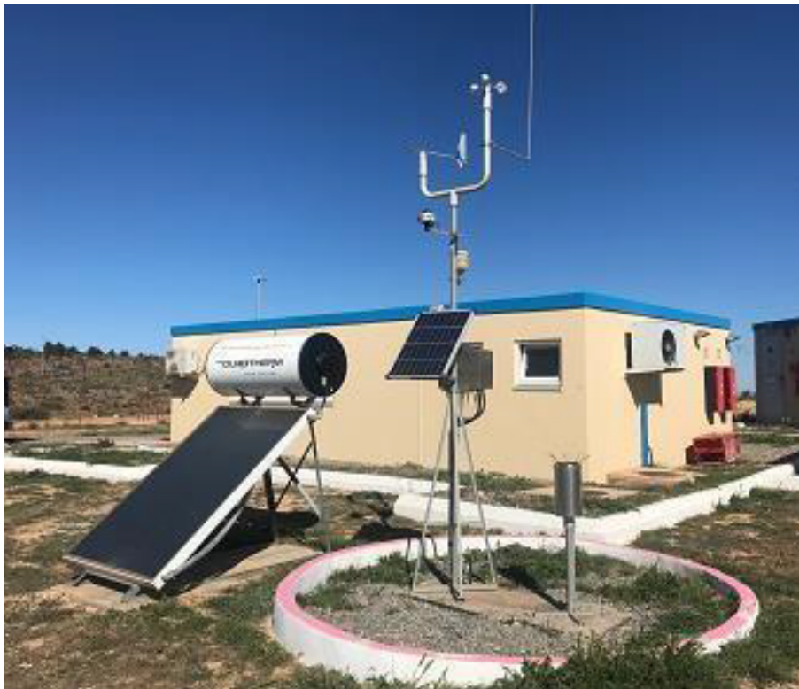
Figure 29. Meteorological mini-station of the Dhaya power plant[59].
