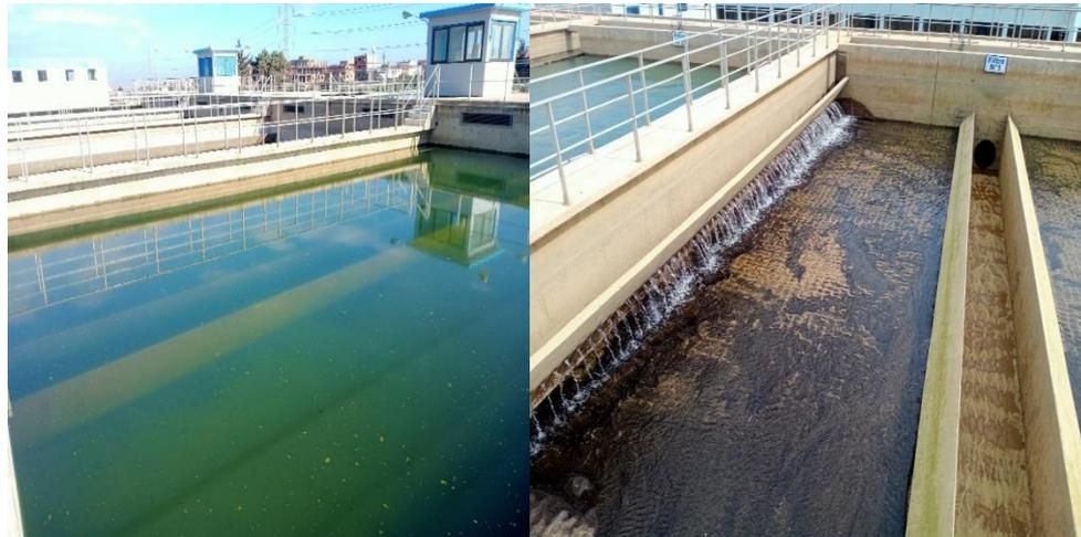
**Figure A.6.**Filtre aquazur type V.
