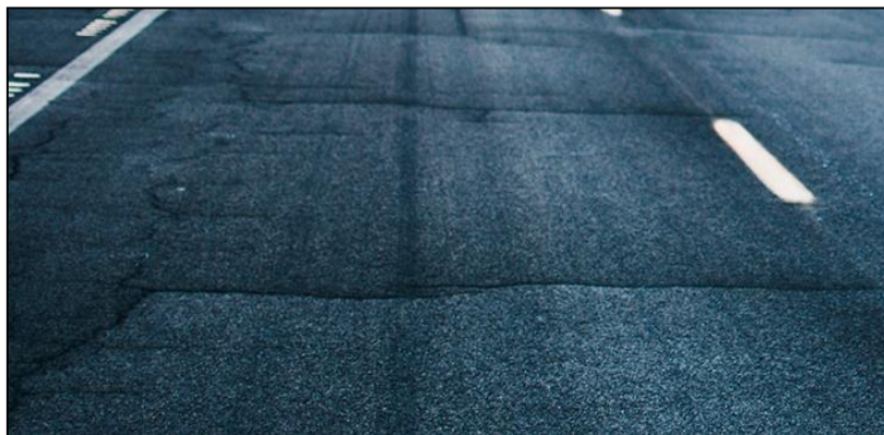
Figure I.17 : Fissures transversales
