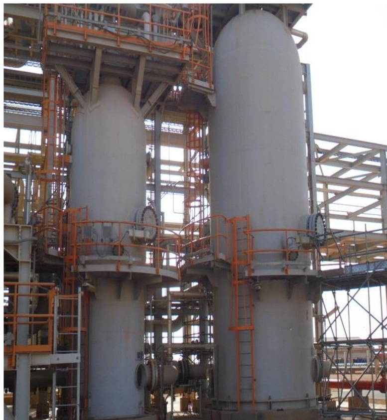
Figure II-5: H 2 S and Hg absorbers.
