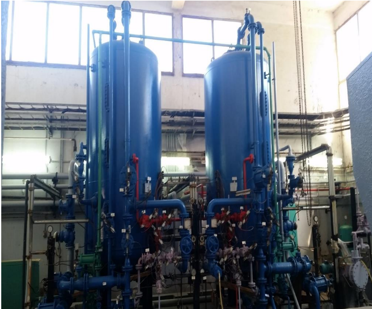
Figure II.1: Mixed Bed Filters
