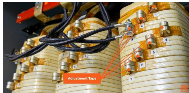
Figure II-12 Power transformer adjustment taps.
