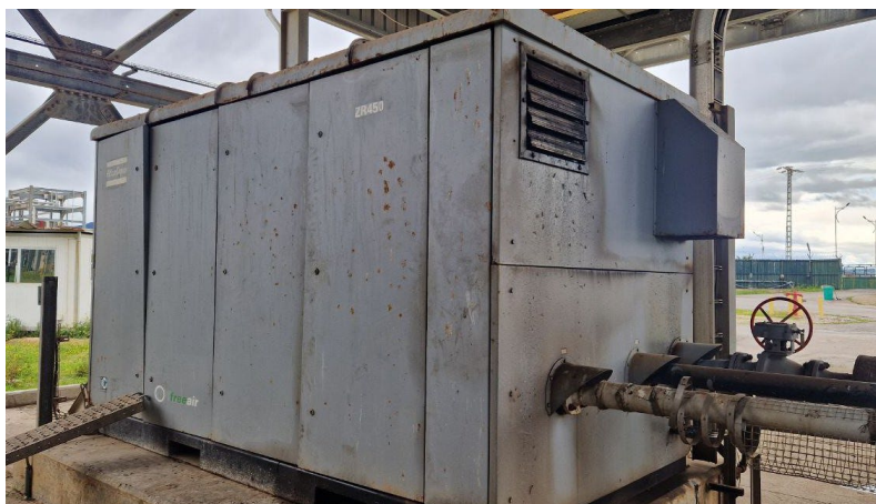
Figure 2.6: Air Compressor Package, 56-MJ01-A/B/C
