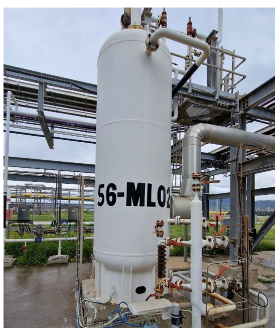
Figure 2.7: Wet Air Separator, 56-ML02
