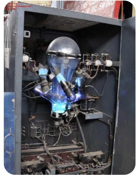
Figure I-2: Mercury arc rectifier under operation [34]
