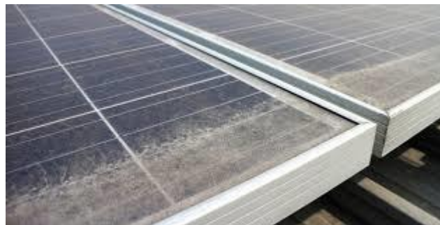
Figure 2.5: Soiling on a PV module
