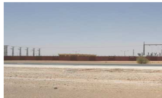
(West side: 30/220kV power station)
