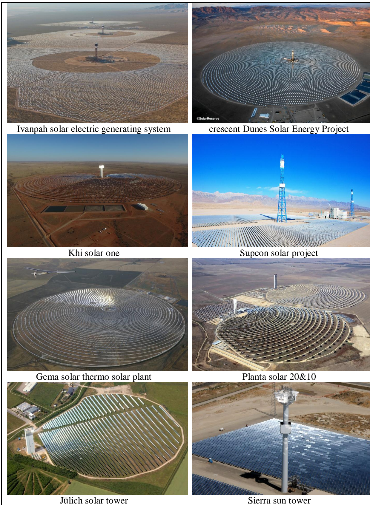
Fig.2.2. Examples of Solar Power Tower Projects [google maps]
