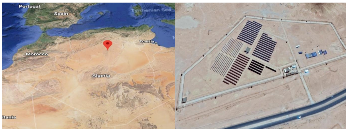
Fig. 1. The geographical situation of Ghardaia city in Algeria's Sahara (on the left), and an overview of the installation of the four grid-connected PV systems (on the right)
