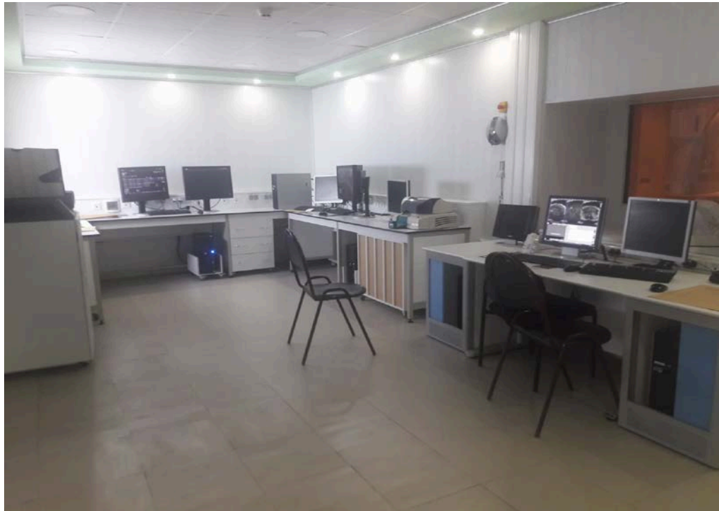
Figure 3.4: Centre de commande.
