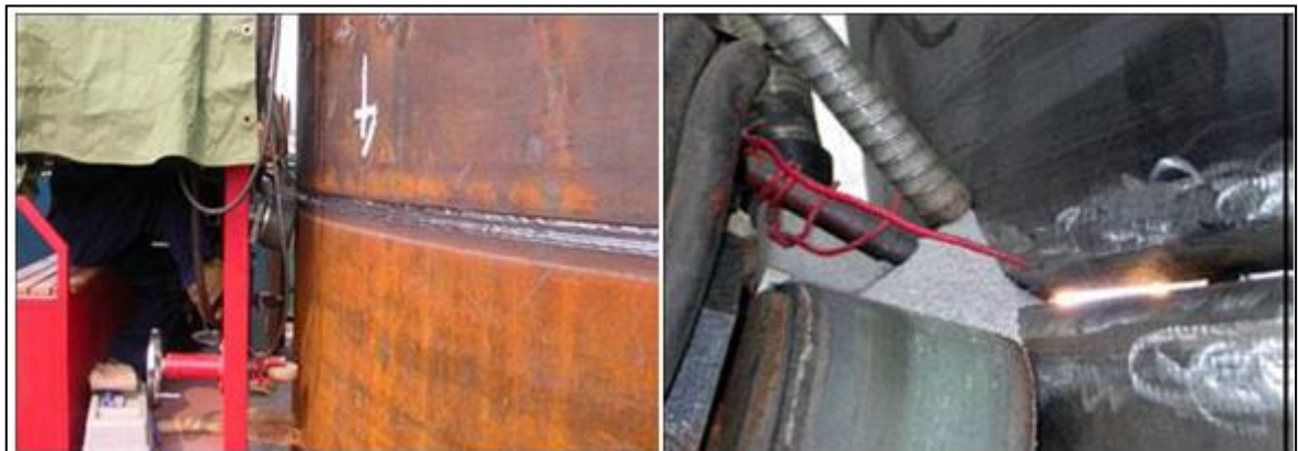
Figure VII. 5 Soudage SAW
