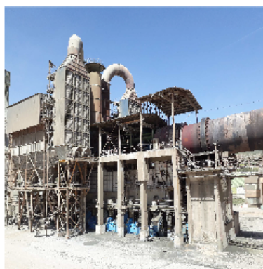
(b) cooler system with its heat exchanger and filter to the left and kiln end appears to the right.
