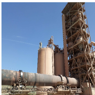
(a) pre-heater tower at the right along with rotary kiln laying in horizontal to the left.
