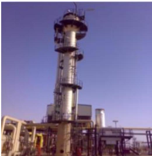
**Figure III.6 :** Stripper C
