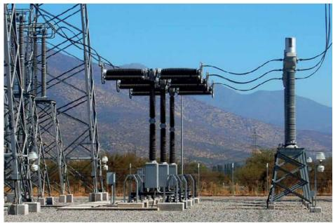
Figure 1.1: High Voltage Circuit Breaker from Siemens
