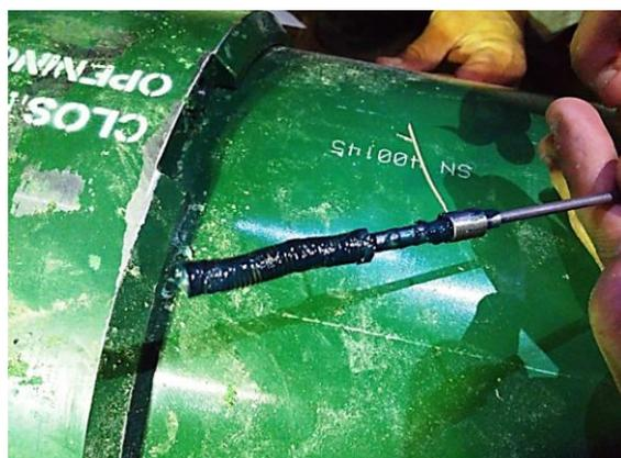
**Fig15: Remove the existing shear pin and install the replacement shear pin (1250psi)**
