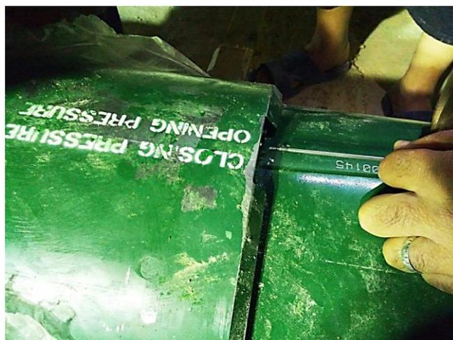
**Fig.20: Remove the closing valve from the valve housing**
