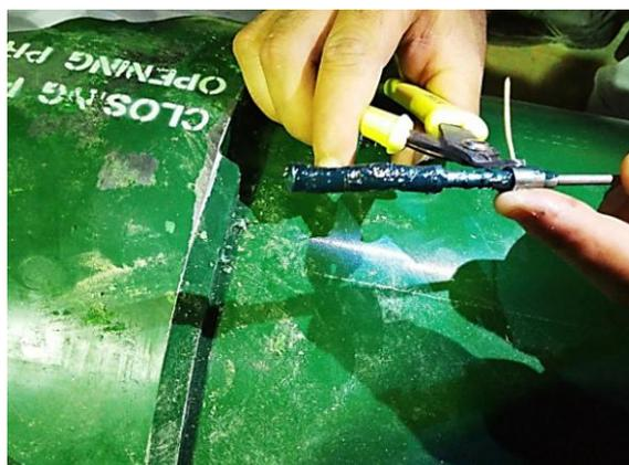
**Fig.16: Cut the replacement shear pin**
