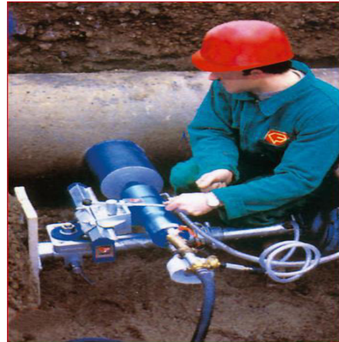
Figure I-7 : Carottage horizontal
