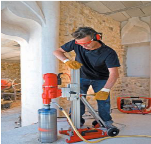
Figure I-6.: Carottage vertical
