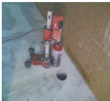
Figure I.15: Carottage [14].
