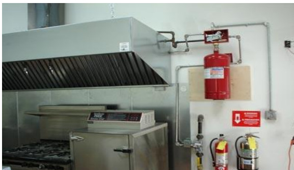
Figure I. 5 Wet chemical system. [20]
