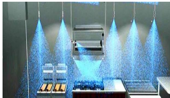
Figure I. 6 Applying wet chemical agent. [21]
