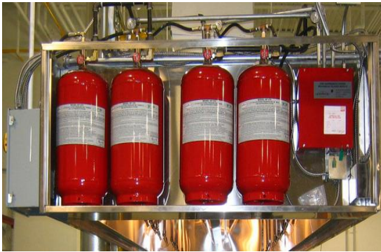
Figure I. 4 Dry chemical system. [16]
