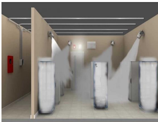
Figure I. 2 Nozzle of a mounted aerosol fire suppression system [14]
