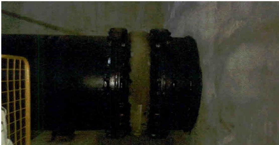
**Figure IV- 8: joint de compensation**
