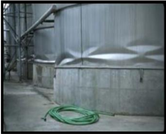
Figure III.9 : Flambement en pointe de diamant (Photos Courtesy of University of California, Brekely)
