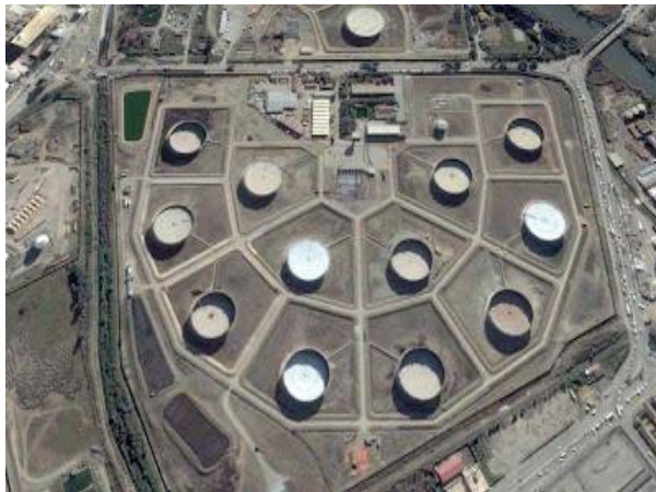
Figure I.6: Terminal nord et sud
