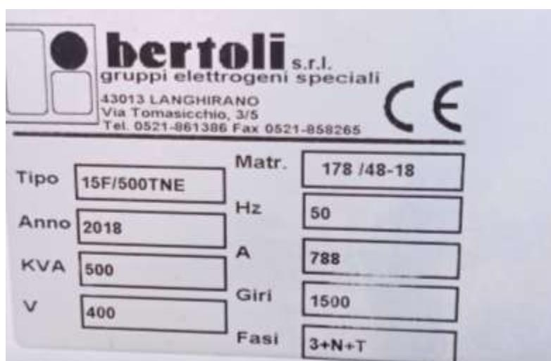
Figure III. 2: plaque signalétique Bertoli 500KVA
