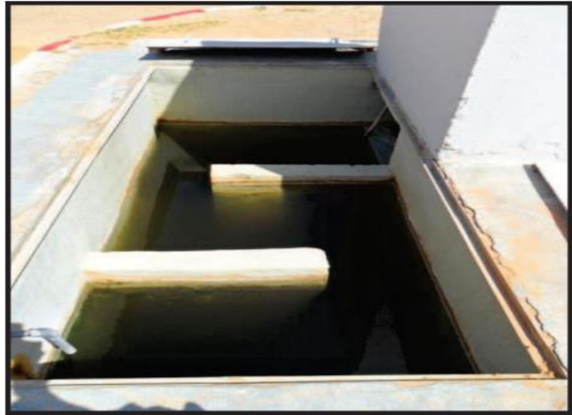
Photo II.6.Bassin de chloration
