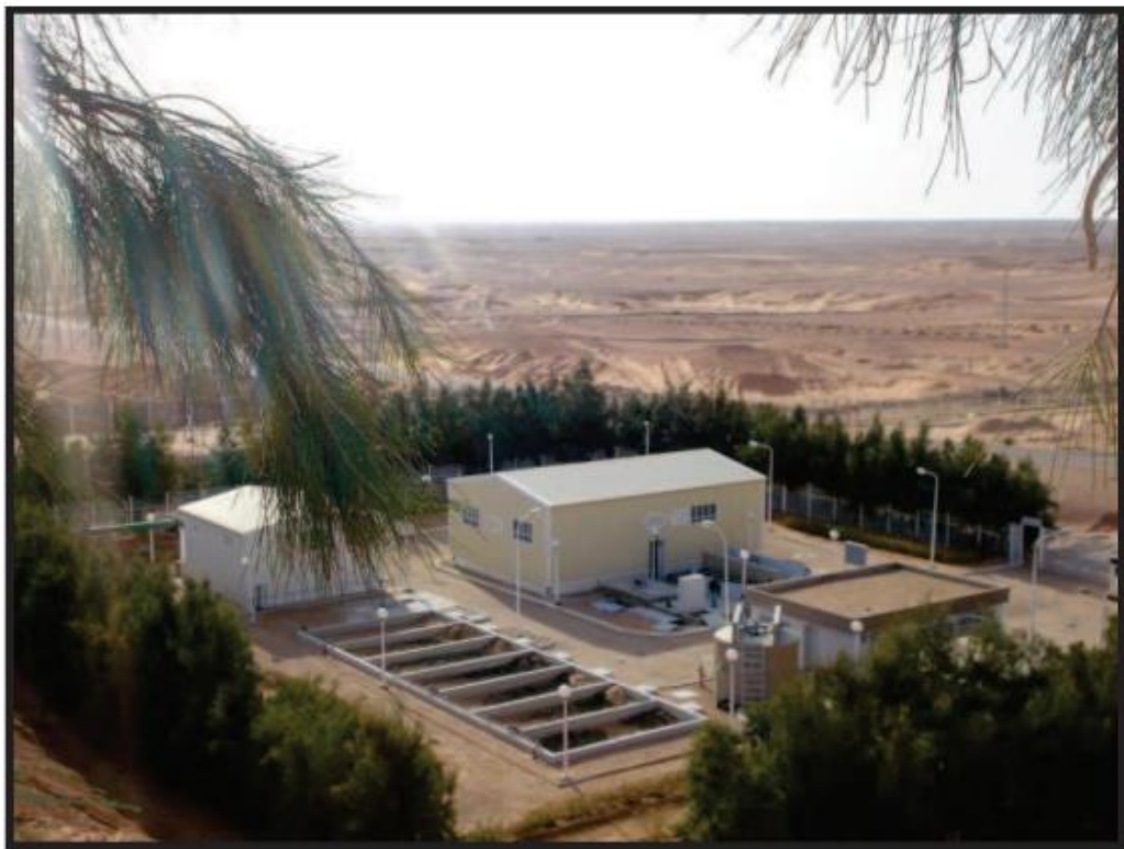
Photo II.1. Station d'épuration HBK
