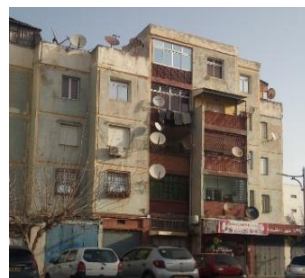
(b) RC wall building in Zone 2 (1983)
