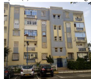
(e) RC wall building in Zone 5 (2010)
