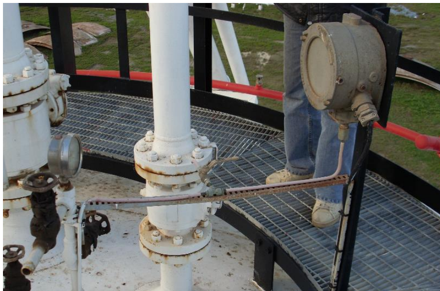
Figure II.17 : Pressostat.
