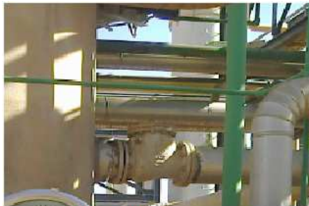
Figure I. 10 Vanne à soupape.
