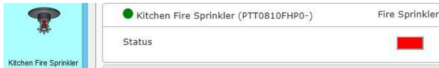
Figure 4.17. The fire sprinkler is OFF.
