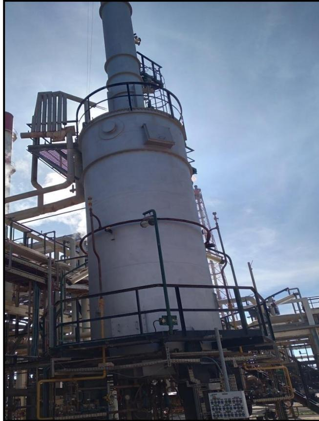
**Figure IV-I-4:** Image correspond au four H201 "cylindrique"
