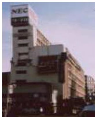
Photo 1.5 : Dissymétrie architectural (oscillations asynchrones) [2], [3]
