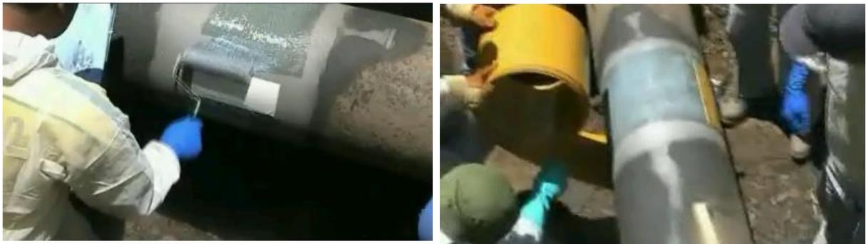
**Figure V. 3:** (1 ;2 ;3 ;4 ;5)Installation de Clock Spring.
