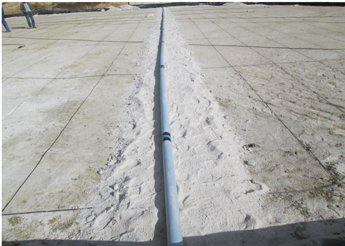
Figure IV. 24 Monitoring tube underneath the tank's bottom surface.
