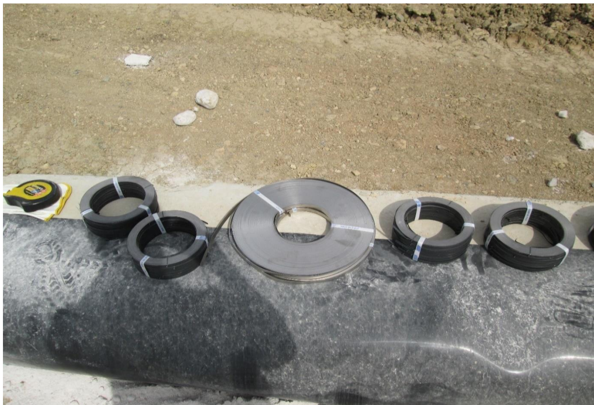
Figure IV. 23 Rolls of ribbon anodes and distribution bars.
