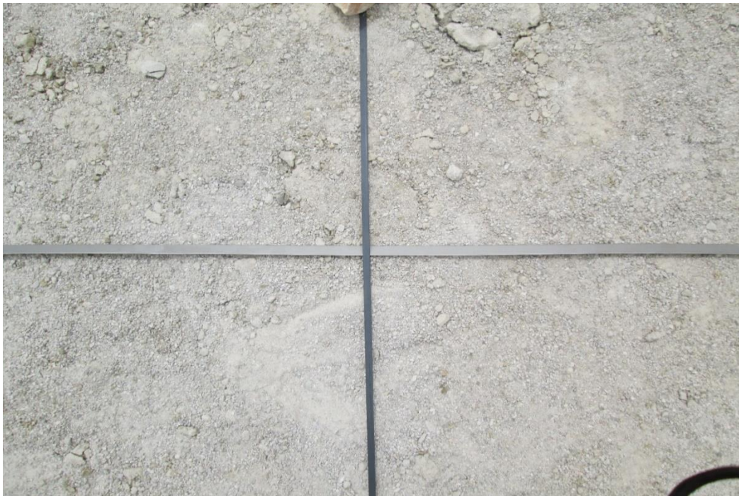
Figure IV. 22 Placement of ribbon anodes on top of the distribution bars.
