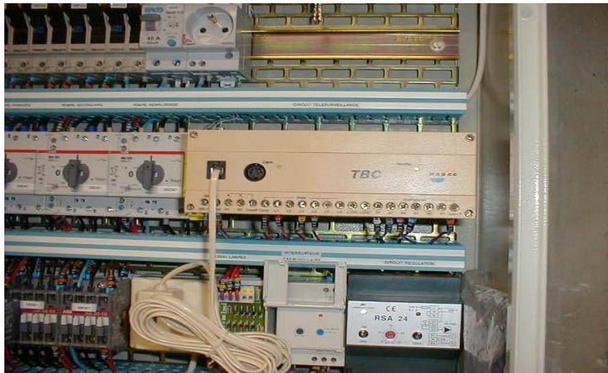
Figure IV.3 LA CENTRALE DE MESURE TBC SOLAIRE
