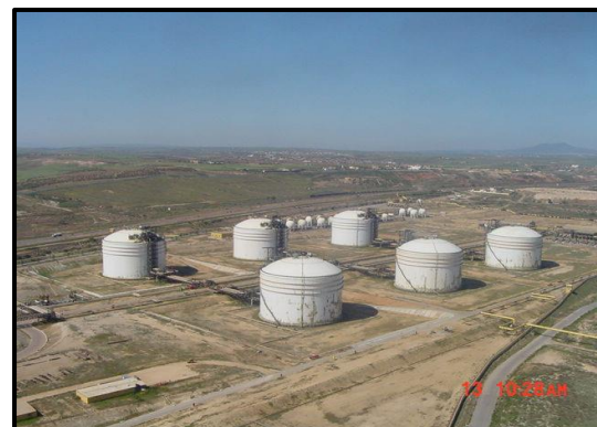
Figure I-16 : Bacs de stockage.
