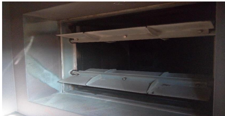
Figure 3-9 : Le registre Four RA2/K
