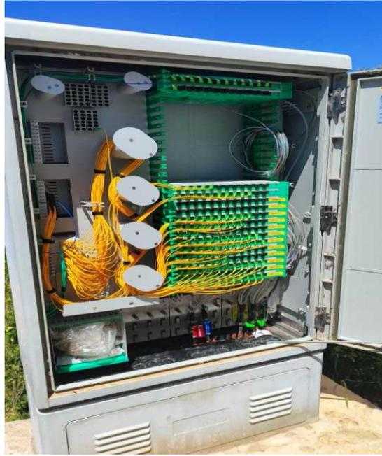
Figure II. 11: FDT (Fiber Distribution Terminal)
