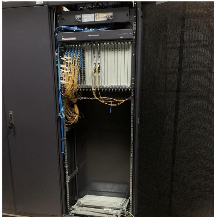
Figure II. 9: OLT (Optical Line Terminal) [17]
