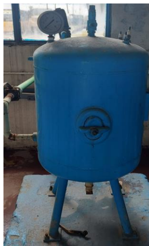
Figure II-7 : Ballon de pression.
